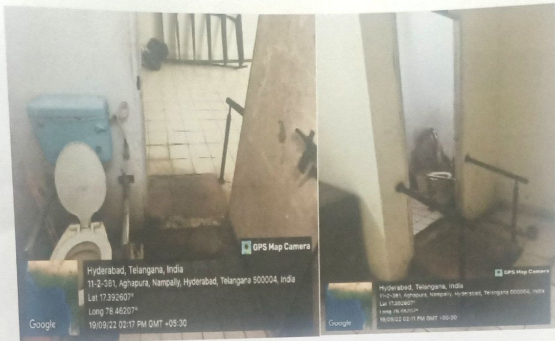
Toilet facilities for Differently-abled
